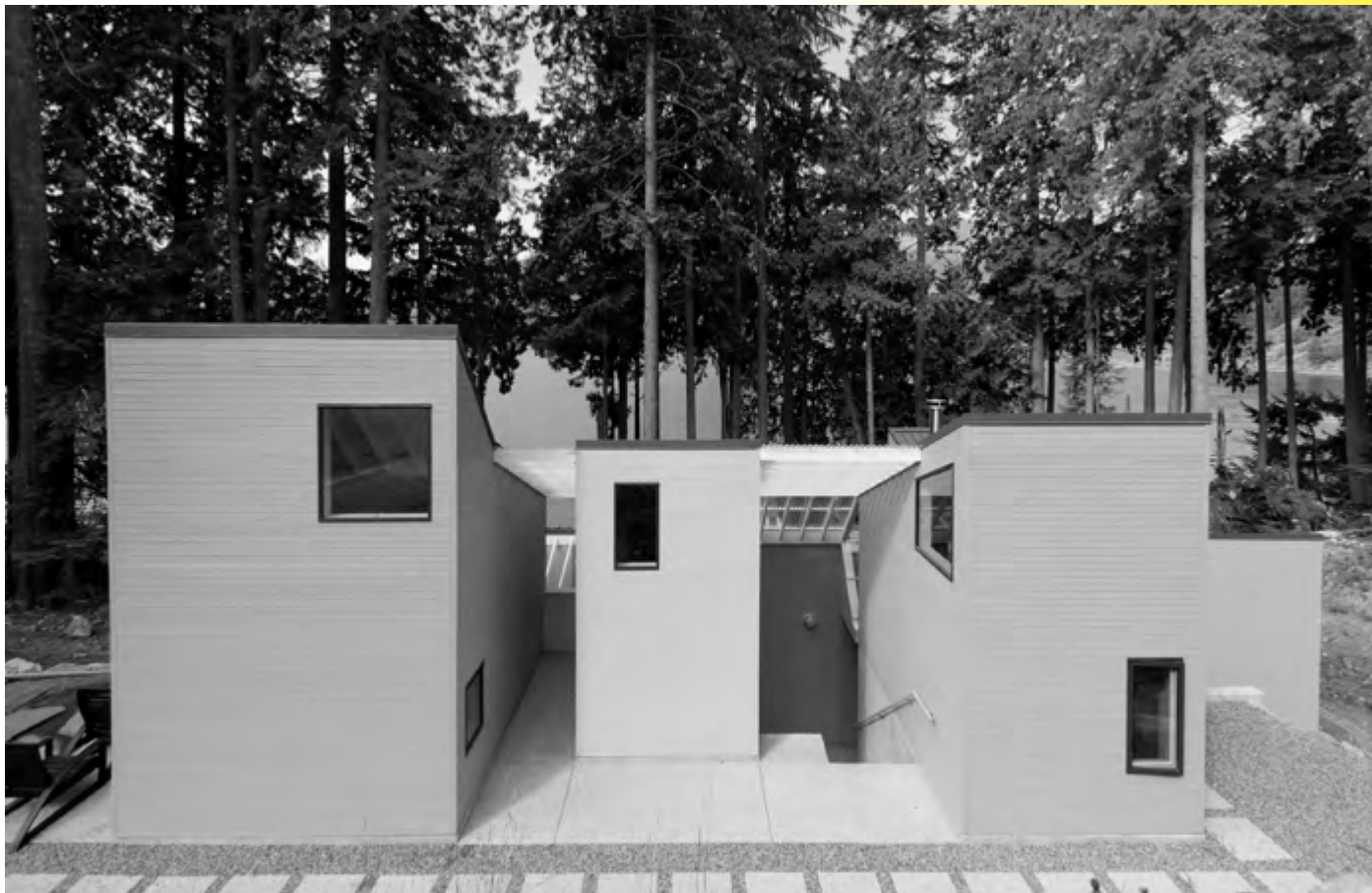
Simcic + Uhrich Architects' Gambier Cabin , Gambier Island
